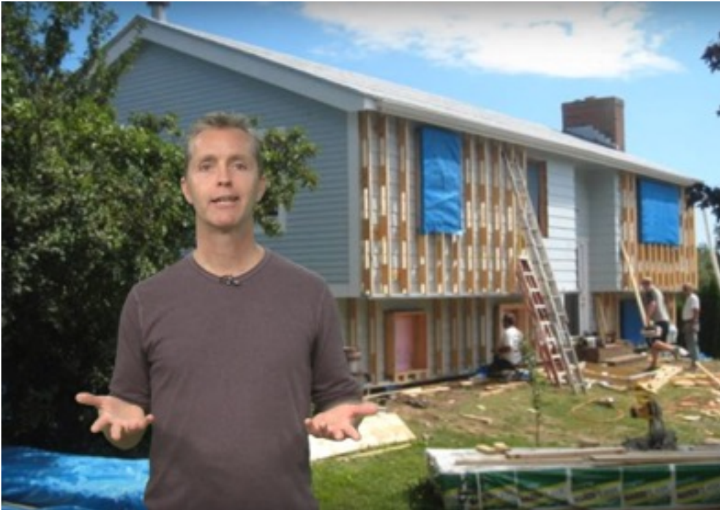
Screen shot from video: House in-progress
